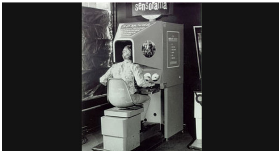
Figure 3: Prototyped in 1956 and patented in 1962, the Sensorama was one of the earliest virtual reality machines. It included full colour 3d video, audio, vibrations, smell, and even wind ( https://virtualspeech.com/blog/history-of-vr )
